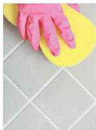
STEP 5 : CLEAN SURFACE AFTER 12 HOURS WITH WATER
